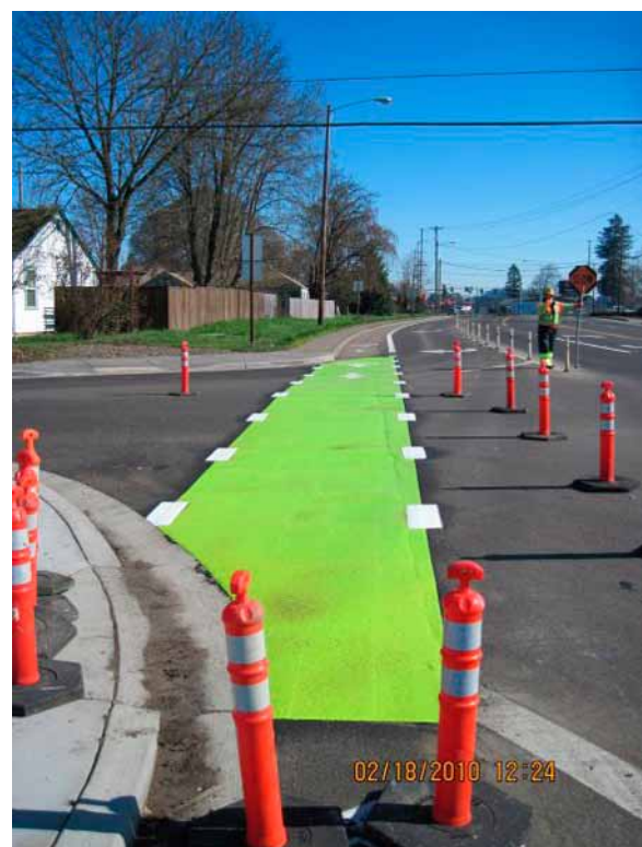
This bike lane in Eugene, OR is painted a bright green at the intersection to increase cyclist safety.
