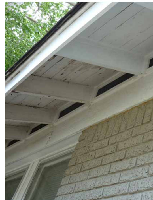
Overhang after fascia vents have been installed.
